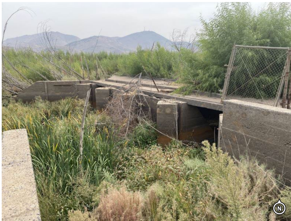
Figure 3-17. Outside of the Canal Inlet Structures
