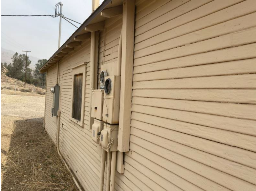
Figure 3-18. Outside of the Storehouse
