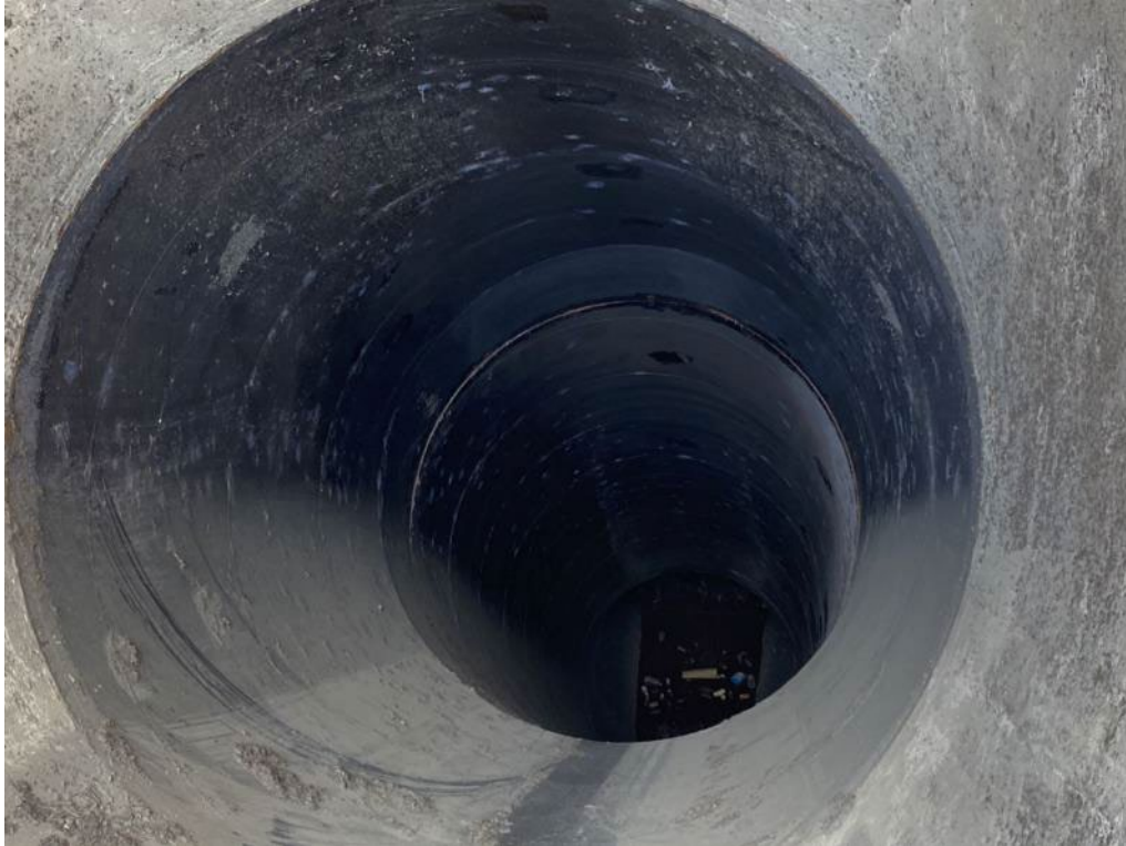
Figure 3-20. Interior of Bodfish Siphon
