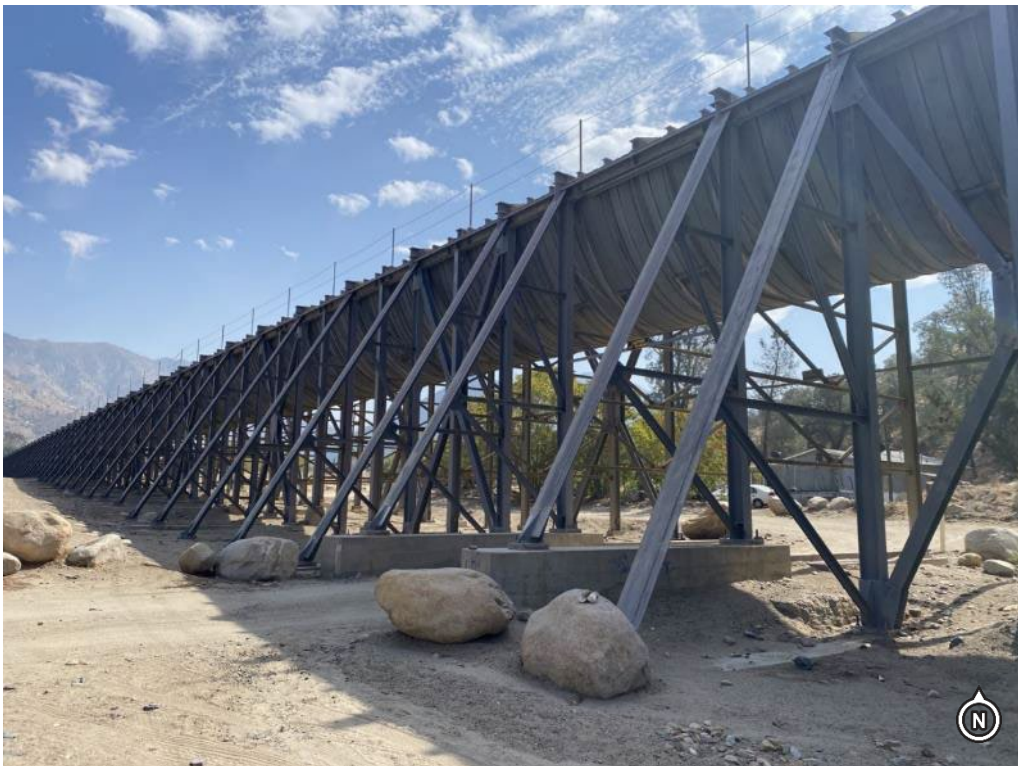
Figure 3-19. Erskine Creek Steel Flume
