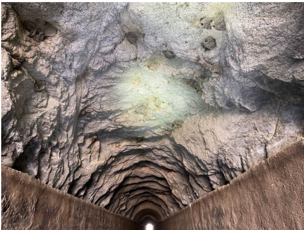
Figure 3-21. Granite Ceiling of Tunnel No. 2
